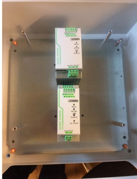
Reinstall middle plate. Remember the earth connections under one of the bolts.
